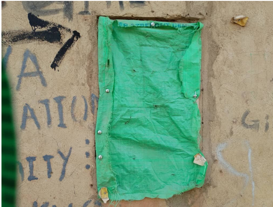
Figure 3: Window covered with a waste cement bag.
