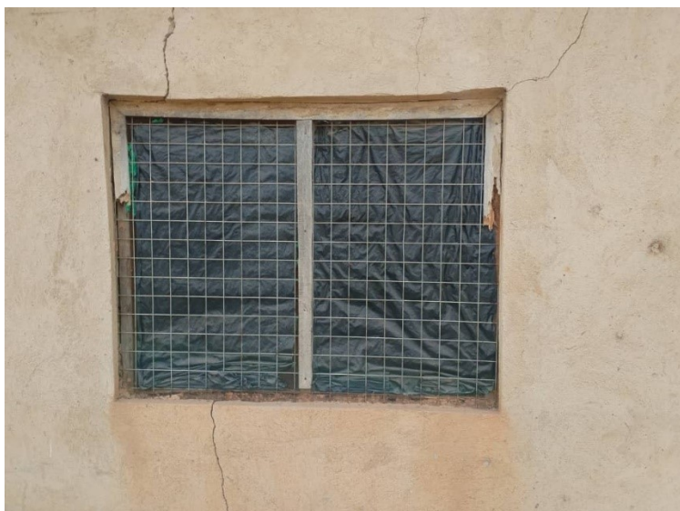
Figure 6: A window completely covered with polythene
