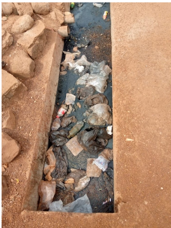
Figure 7: A choked gutter.
