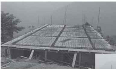
Floor/roof ready for concreting after shuttering and reinforcement placing
