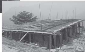
Floor/roof ready for concreting after shuttering and reinforcement placing
