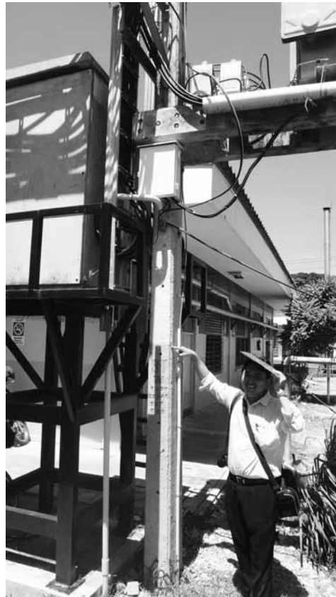
Dr. Komchit Chavanasporn, member of HOPE Assessment team, inspects the elevated electrical circuit board which was raised to a higher level after flooding which hit Ayutthaya Hospital
