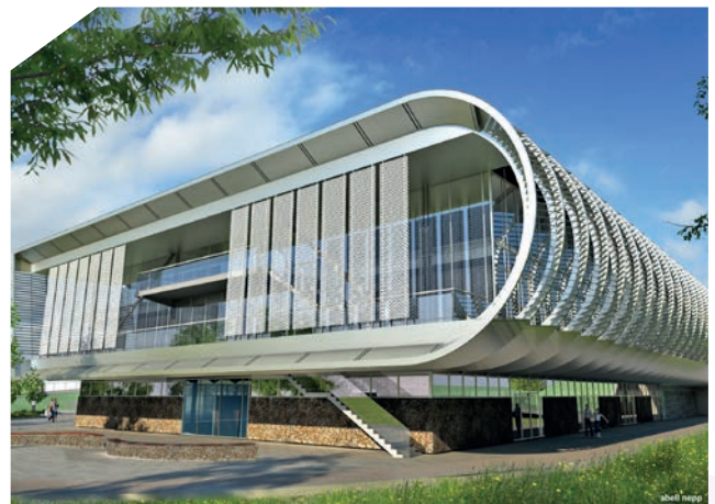
D4FC: Technical Hub at EBI, Cambridge, showing detailed solution for reducing solar gain / glare (Aecom)
