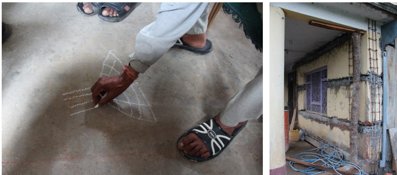
Figure 12. A mason in Bhaktapur drew how they now bent reinforcing steel into foundation footing, rather than simply cutting them at the foundation. The mason explained that he learned this technique as part of his school retrofit training. In North Kathmandu, houses near the school retrofit site were being retrofitted by adding bands and stitches two months after the event. The work was being carried out by local masons who had been trained to retrofit the school. Photo: R. Paci-Green/Risk RED
