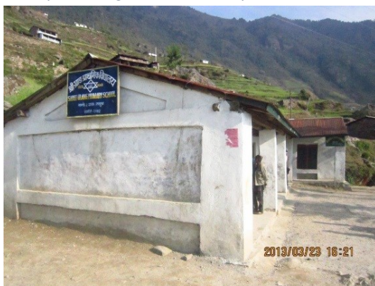
Figure 6. Donor-funded retrofit of a stone and mud mortar school in Rasuwa collapsed in the earthquake, as the principal captured and showed us on his smart phone after retrofit on the left and after the earthquake on the right. The rubble had been removed by the time of the survey. Little training of masons and nearly non-existent technical oversight ensured that when masons struggled to implement the retrofit design, the problems were not caught and rectified. The principal estimates 120 out of 140 students and staff would have died. Photos courtesy of school principal.
