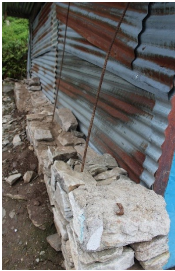
Figure 4. A Ministry of Education template design, which called for vertical rebar to be placed in stone walls, completely collapsed in every block assessed with this design. While now removed, after the earthquake, the classrooms were filled with stone from the collapsed walls. Photo: R. Paci-Green/Risk RED
