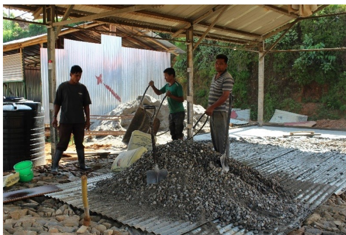
Figure 14. Untrained masons are already rebuilding school buildings without incorporating disaster-resistant construction techniques. The masons here were not measuring concrete materials accurately and were using only large aggregate in their mixture. When asked, the masons said that they learned to lay reinforcing steel bars shown from previous metal frame school construction. They were incorrectly laying rebar on the ground, without spacers, and without bar end hooks. The school buildings of which they spoke had collapsed or been badly damaged. Photo: R. Paci-Green/Risk RED
