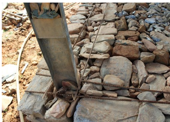
Figure 14. Untrained masons are already rebuilding school buildings without incorporating disaster-resistant construction techniques. The masons here were not measuring concrete materials accurately and were using only large aggregate in their mixture. When asked, the masons said that they learned to lay reinforcing steel bars shown from previous metal frame school construction. They were incorrectly laying rebar on the ground, without spacers, and without bar end hooks. The school buildings of which they spoke had collapsed or been badly damaged. Photo: R. Paci-Green/Risk RED
