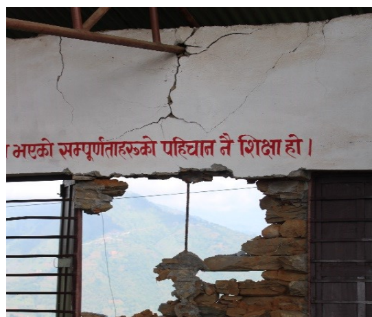
Figure 7. This teaching resource centre on school grounds was built with stone and mud mortar. The masons employed earthquake-safety measures, such as a reinforced concrete lintel band and vertical reinforcement in the walls. However, even with these measures, the heavy shaking in Sindhupalchowk caused the stone building to collapse swiftly and completely. It may be difficult to rebuild safe schools out of this brittle material unless alternative technologies are developed, tested and extensive mason training and strict oversight are feasible during construction. Photo: R. Paci-Green/Risk RED
