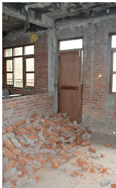
Figure 2. School building 101-1, which experienced only moderate shaking in Bhaktapur, was deemed unsafe for school use because unreinforced partition walls separated from the reinforced concrete frame and became unstable. Damage to unreinforced partition or infill walls can injure or kill students and block exits. The safety of these walls is routinely ignored by engineers and communities alike. Photo: R. Paci-Green/Risk RED
