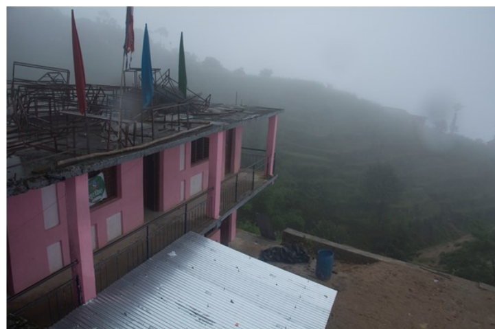
Figure 5. While a retrofitted school in Kathmandu performed well in this earthquake, retrofit design and construction flaws may lead to unnecessary damage in larger events. In the left photo, vertical bars poke out the bottom of a retrofit band. A horizontal retrofit band at the bottom of the wall is missing on this side of the building. On the roof top, the vertical bars are secured by only small patches of concrete, partially covered in the photo by discarded school benches. The masonry columns supporting the roof overhang were not strengthened in any way and remain unsupported below the balcony overhang. Photo: B. Pandey/Risk RED
