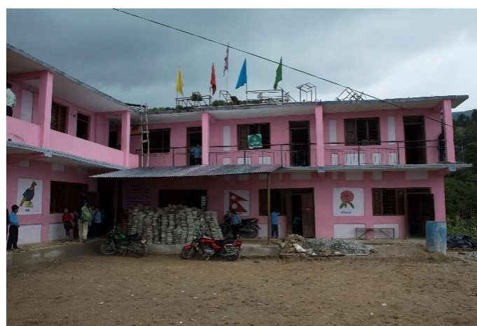
Figure 13. Both schools shown here were successful safer school projects – a new masonry building with lintel and sill bands on the left, and a retrofitted masonry building on the right. Neither provides highly visible signage to alert communities of the safer construction techniques employed, though the school on the left did paint a safe evacuation plan on the building. The lintel and sill bands are barely visible under the white paint in the left photo. The retrofit bands are highlighted in bright pink in the photo on the right, but could have been labelled as earthquake-resistant retrofit bands for an ongoing reminder of the project and of the community's exposure to earthquake risk. Photo left: R. Paci-Green/Risk RED. Photo right: R. Friedman/Risk RED
