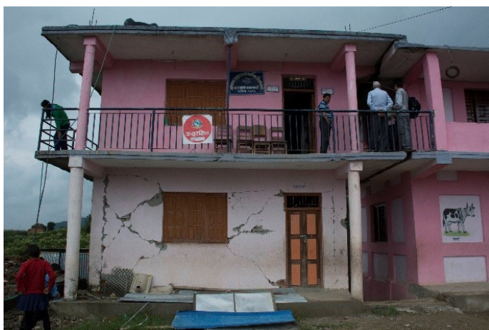
Figure 1. At a school in Kathmandu, two school buildings on the same sight performed very differently. The building on the left, a reinforced concrete frame structure with brick infill walls, was moderately damaged and received a red tag. Its frame joints and infill walls will need to be repaired before the building can be reused for classrooms. The building on the right, an adobe and stone masonry structure, was recently retrofitted with stitch banding. It was undamaged and immediately able to be reopened, despite being made of a weaker building material. The retrofit proved to be successful. Photo: R. Friedman/ Risk RED
