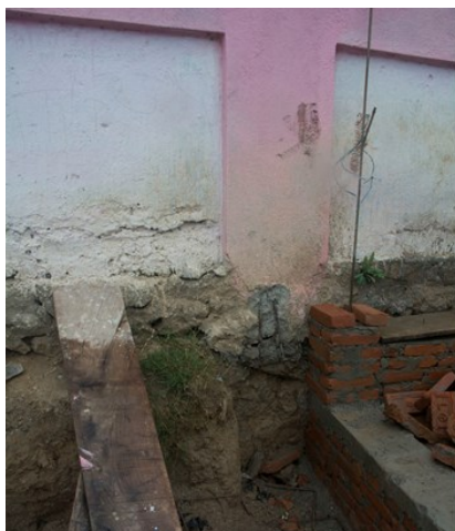
Figure 5. While a retrofitted school in Kathmandu performed well in this earthquake, retrofit design and construction flaws may lead to unnecessary damage in larger events. In the left photo, vertical bars poke out the bottom of a retrofit band. A horizontal retrofit band at the bottom of the wall is missing on this side of the building. On the roof top, the vertical bars are secured by only small patches of concrete, partially covered in the photo by discarded school benches. The masonry columns supporting the roof overhang were not strengthened in any way and remain unsupported below the balcony overhang. Photo: B. Pandey/Risk RED
