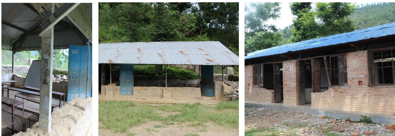
Figure 3. Metal frame template designs are common in rural and remote areas. While the frames were undamaged in the earthquake, the stone and mud mortar walls that used to enclose the school collapsed. These walls were considered non-structural. Communities were allowed to build them with available materials and without reinforcement. The vast majority of the stone walls collapsed down to about half a meter, showering the classroom with large, deadly stones. Brick walls were typically damaged and unstable, but collapsed less often. [Note: Rubble from collapsed stone and brick had already been removed when photos were taken.] Photo: R. Paci-Green/Risk RED
