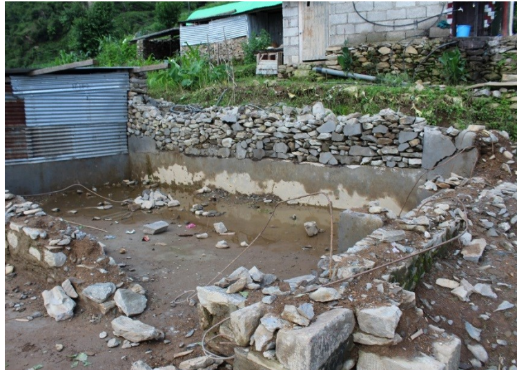
Figure 4. A Ministry of Education template design, which called for vertical rebar to be placed in stone walls, completely collapsed in every block assessed with this design. While now removed, after the earthquake, the classrooms were filled with stone from the collapsed walls. Photo: R. Paci-Green/Risk RED
