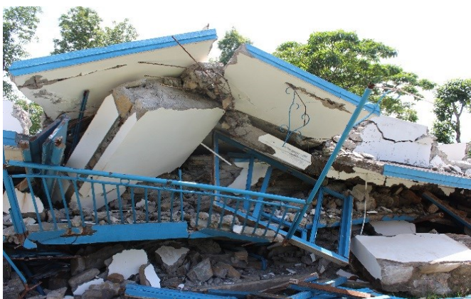
Figure 8. Two neighbouring schools were both built through international donor support. The left was built without technical support. The right was built after the community was given an orientation on earthquake safe construction and local masons were trained in safer construction techniques. An engineer and lead mason, both with experience in earthquake-safe school construction, carefully oversaw the process. After the earthquake, the second was operational; even the terrace had been covered and converted into a makeshift workshop for the local community. Photo: R. Paci-Green/Risk RED
