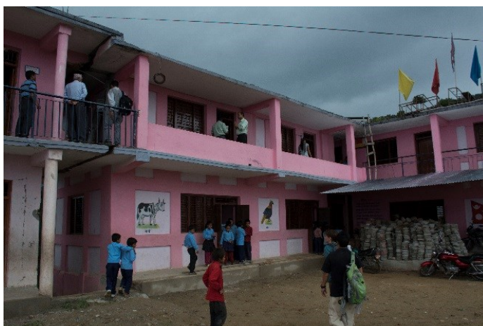
Figure 1. At a school in Kathmandu, two school buildings on the same sight performed very differently. The building on the left, a reinforced concrete frame structure with brick infill walls, was moderately damaged and received a red tag. Its frame joints and infill walls will need to be repaired before the building can be reused for classrooms. The building on the right, an adobe and stone masonry structure, was recently retrofitted with stitch banding. It was undamaged and immediately able to be reopened, despite being made of a weaker building material. The retrofit proved to be successful. Photo: R. Friedman/ Risk RED
