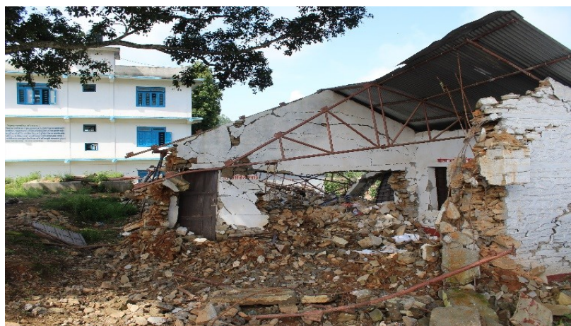
Figure 7. This teaching resource centre on school grounds was built with stone and mud mortar. The masons employed earthquake-safety measures, such as a reinforced concrete lintel band and vertical reinforcement in the walls. However, even with these measures, the heavy shaking in Sindhupalchowk caused the stone building to collapse swiftly and completely. It may be difficult to rebuild safe schools out of this brittle material unless alternative technologies are developed, tested and extensive mason training and strict oversight are feasible during construction. Photo: R. Paci-Green/Risk RED
