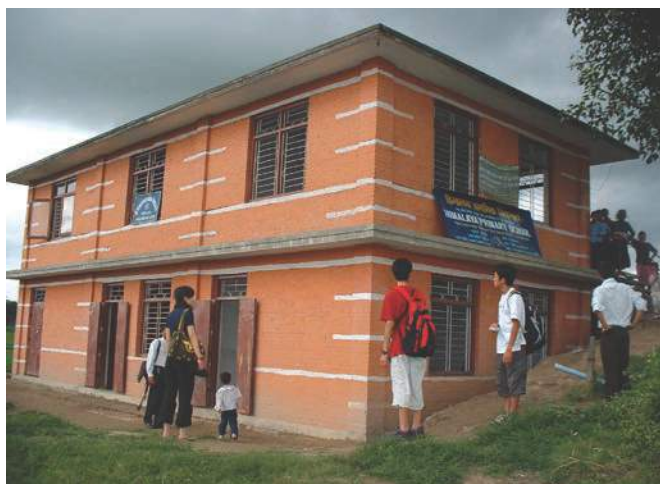
Reinforced concrete bands in a masonry school building are highlighted with bright white marks in Nepal. Parents now use these techniques in the construction of their own homes. Traditionally, the community built masonry houses without reinforcement. Photo: Bishnu Pandey.
