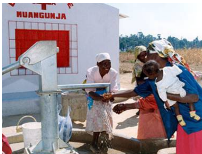
Angola New water point at a Red Cross clinic
