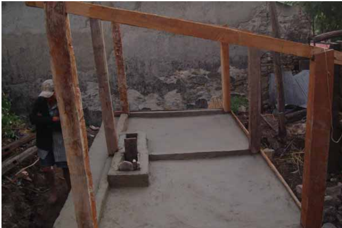
A model pigsty under construction
