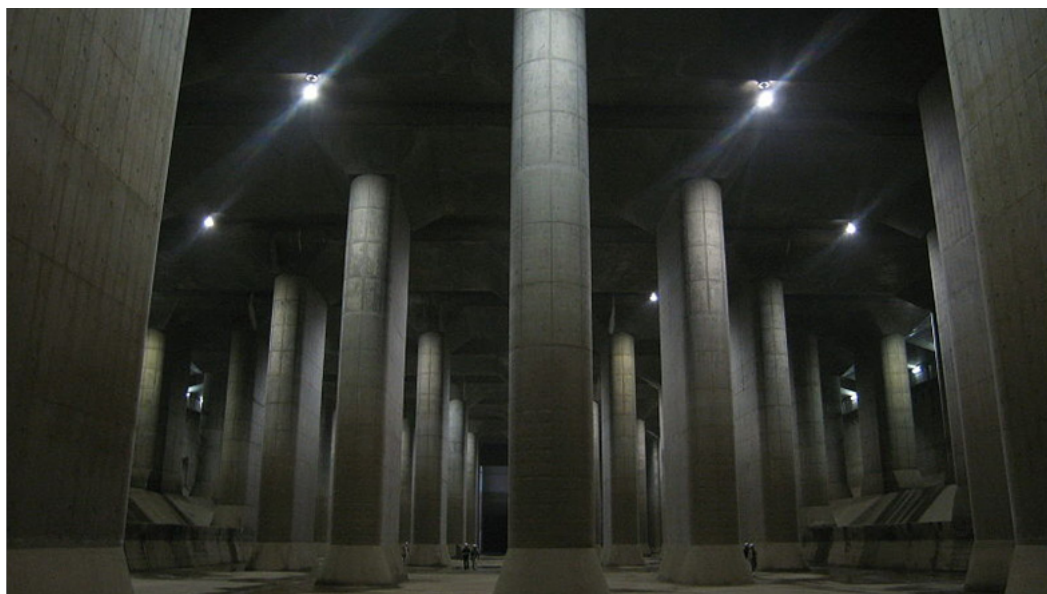
The Metropolitan Area Outer Underground Discharge Channel, also known as the G-Cans Project, is an underground water infrastructure project in Kasukabe, Saitama, Japan. It is the world's largest underground flood water diversion facility, built for preventing overflow of the city's major waterways and rivers during rain and typhoon seasons. Photo credits: Adapted from the Wikimedia Commons: http://commons.wikimedia.org/wiki/File:Kasukabe2006_06_07.JPG by Dddec0
