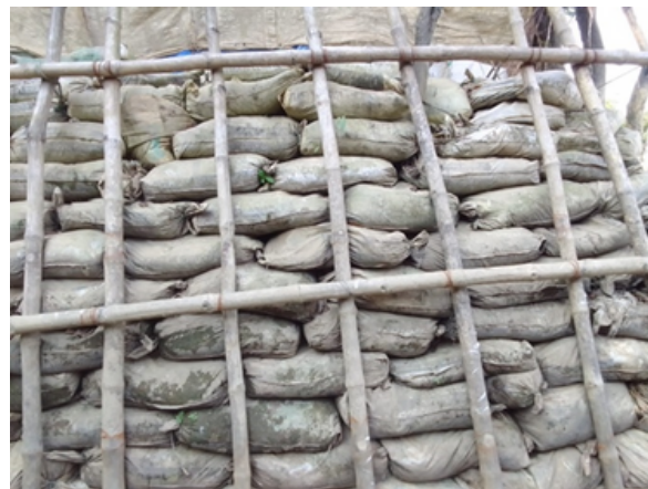
Raising the plinth level of houses is a common flood preparation action in the community. During the dry season, soil is collected from riverbeds to elevate homes, with bamboo sticks or sand-filled cement bags used to prevent erosion from wave action. Wealthier residents may use CC blocks or bricks for added protection.
