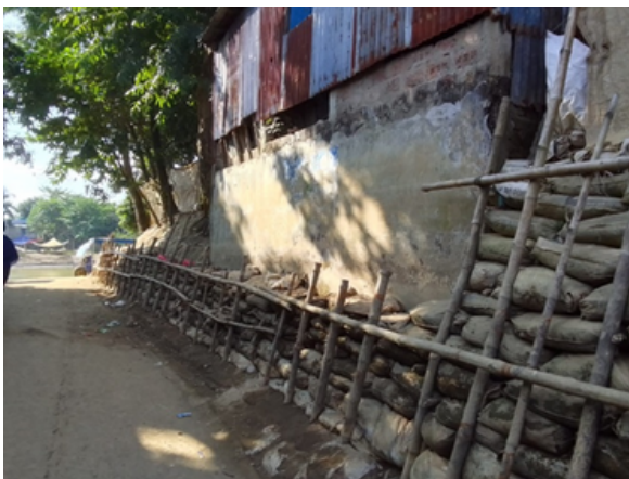
Raising the plinth level of houses is a common flood preparation action in the community. During the dry season, soil is collected from riverbeds to elevate homes, with bamboo sticks or sand-filled cement bags used to prevent erosion from wave action. Wealthier residents may use CC blocks or bricks for added protection.
