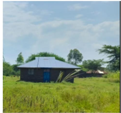
Image 3: A house constructed using iron sheets. Due to the perennial floods, iron sheets are the more preferred housing material used for construction since it can withstand the floods compared to houses made from mud (picture on right hand side).
