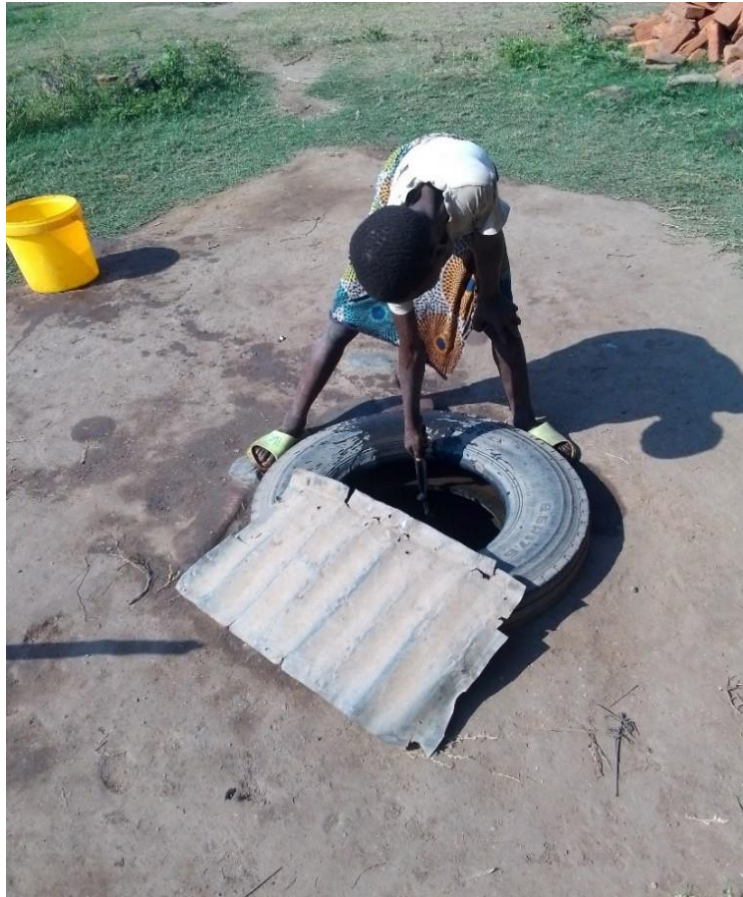
Figure 8: An open well used for drinking water, where a household lacked resources to build a proper barrier and cover, using only a tire, which was insufficient to prevent water from entering during Cyclone Freddy (Photo by the author)
