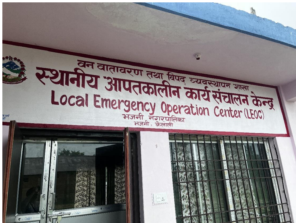
Local Emergency Operations Center in Bhajani Municipality, Kailali.
