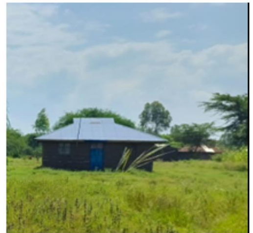
Image 3: A house constructed using iron sheets. Due to the perennial floods, iron sheets are the more preferred housing material used for construction since it can withstand the floods compared to houses made from mud (picture on right hand side).
