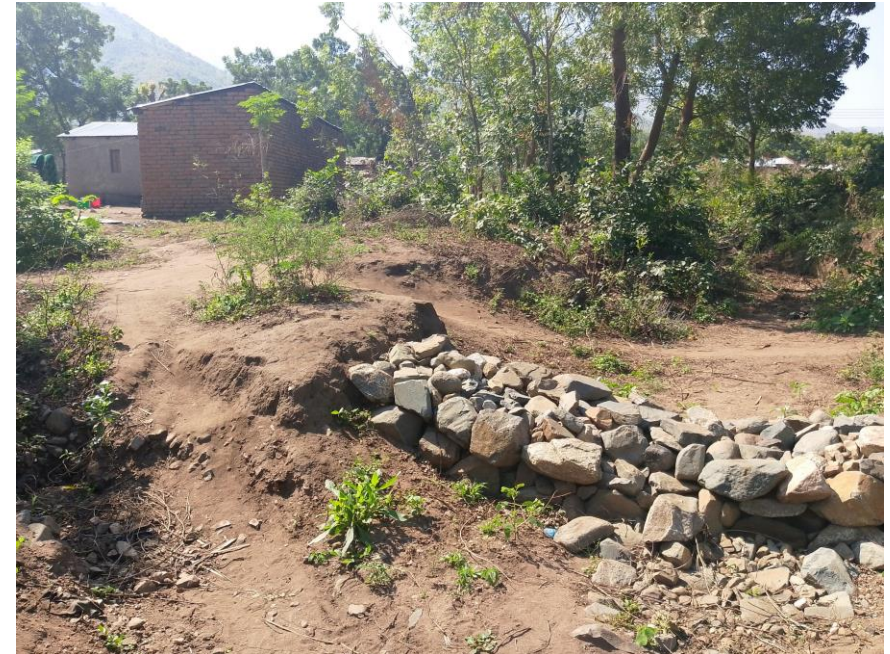
A household in Makhuwira protects its house by constructing a floodwater barrier well ahead of flooding (Photo: fieldwork)
