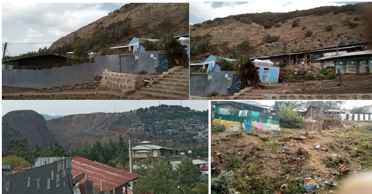
Figure 14: Settlement in the buffer zone (Highly susceptible to landslides and flooding)
